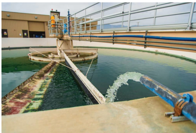
CVWD's WRP-4 has a secondary treatment capacity of 9.9 mgd (11,090 AFY) and has a planned tertiary expansion.
