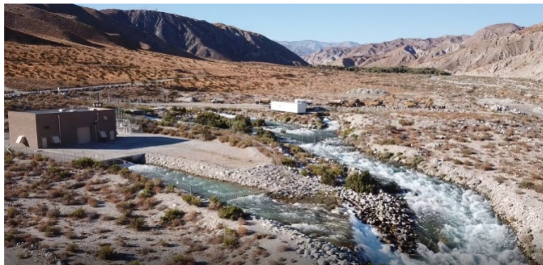
Water from the Colorado River Aqueduct is conveyed through the Whitewater Hydropower Plant and ultimately feeds WWR-GRF.
