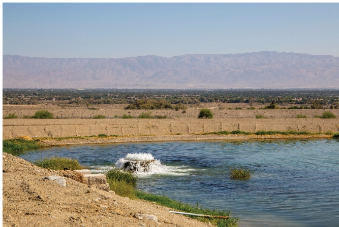
TEL-GRF utilizes a narrow mountain-front forebay for artificial recharge.
