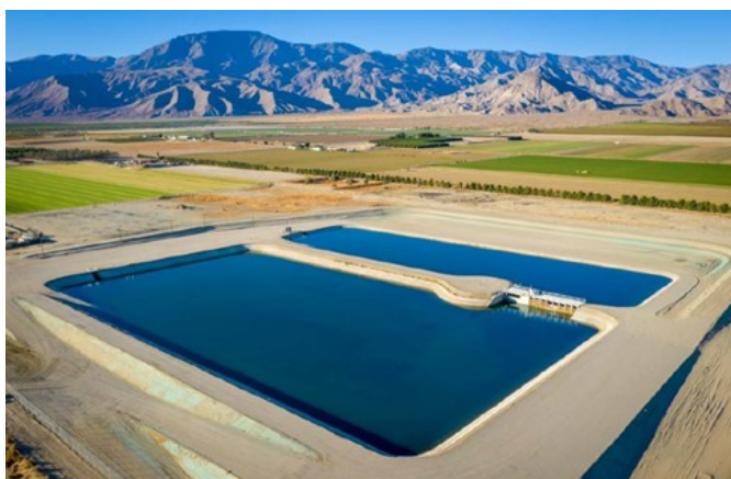
The Oasis Distribution System would further expand the Canal water delivery system to the Oasis Area.
