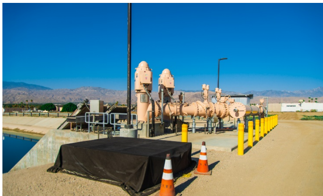
The PD-GRF Expansion will expand direct replenishment capacity at PD-GRF.
