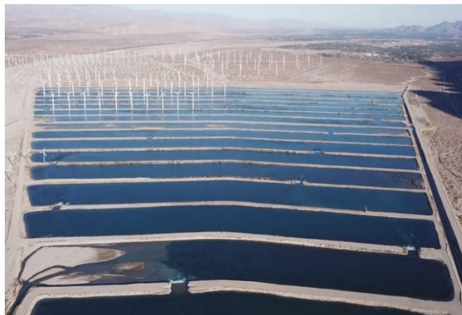
SWP exchange water is recharged at the WWR-GRF.
