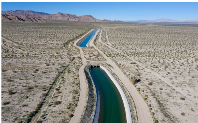
The Colorado River Aqueduct conveys water to the western portion of the Indio Subbasin at the WWR-GRF.
